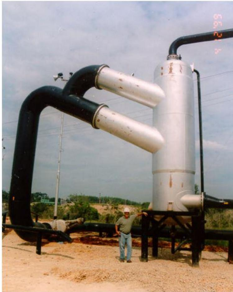
Figure 2-7 GLCC application in a bulk separation/metering loop [17]
