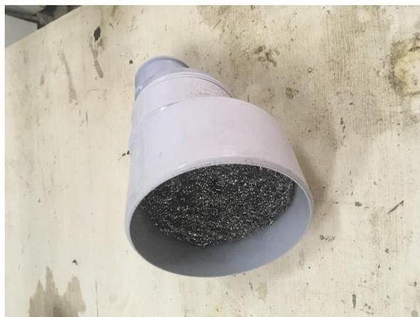
Figure 3-9 Liquid trap
